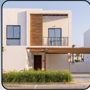
Ready to Build Homes
